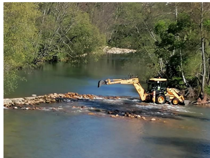
Dams selected for removal
