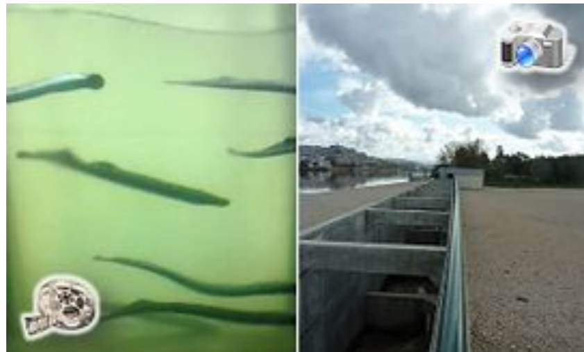
Vertical-slot fish pass in Coimbra Dam
