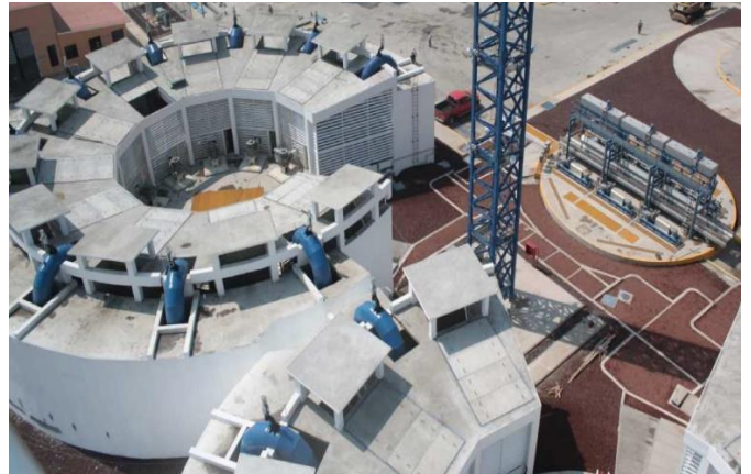
Figure 14. Station de pompage Casa Colorada Profunda.
